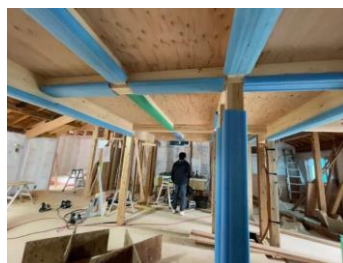
ロフト部分の下側
